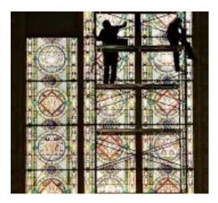
After approximately a month, the repaired glass panel was reinstalled, and the next set of square panels were removed to repeat the process.
