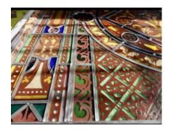
Broken pieces were cut and paint colors were mixed to match the exact color of the original. The paint was then applied to the new section of glass to match the pattern and design of the original. Firing the glass bonded the paint to the glass.
