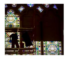
During the five-year restoration of our windows, the scaffolding was set up, square window sections were removed, and painted plywood was placed into the spaces where glass was removed. Huge glass panels were then taken to a studio and each section was taken apart.
